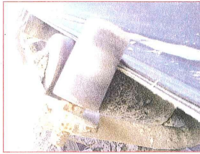
Figure 9. Seized trough trainer, causing ply separation and edge damage to the conveyor belt.
